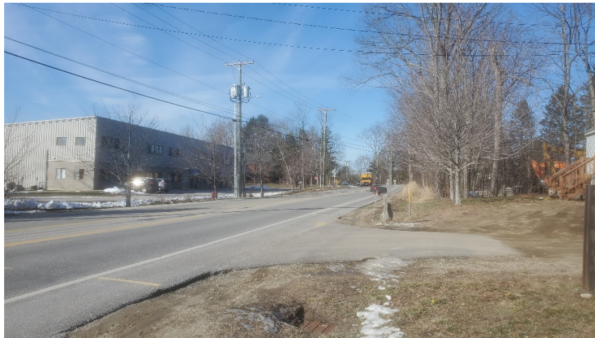
SIGHT DISTANCE LOOKING NORTHERLY
