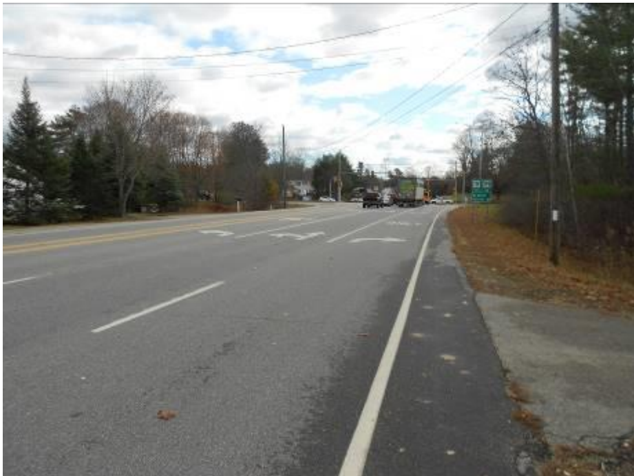
Street Scene – Front of the Subject Property Looking Southeast on Littleworth Road - (11/20)
