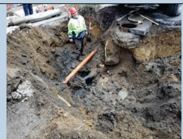
Mill Street Excavation
