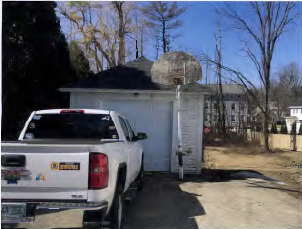
Existing Garage to be Removed
