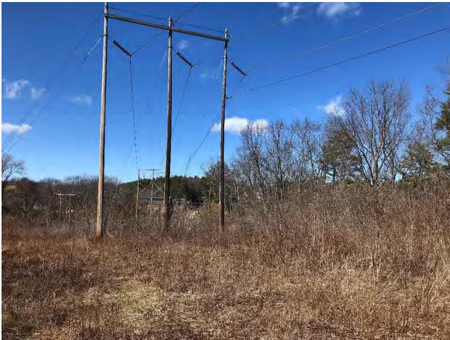
Photograph No. 16: Looking easterly at M183 Structure 86 to be replaced.
