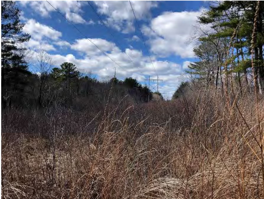
Photograph No. 1: Looking westerly at Wetland DOW-32.2 toward M183 Structure 28 to be replaced.
