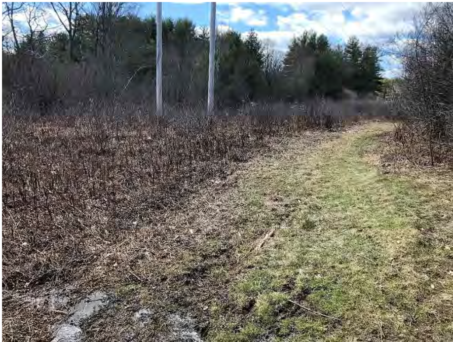
Photograph No. 4: Looking westerly at Wetland DOW-32.3 and M183 Structure 29 to be replaced. Timber matting will be used in the wetland portion of the access and work pad.
