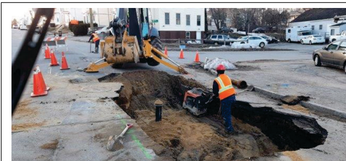
Crew back filling the water main on Ham St.
