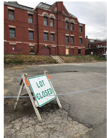
First Street parking lot which will become parking for new apartments.
