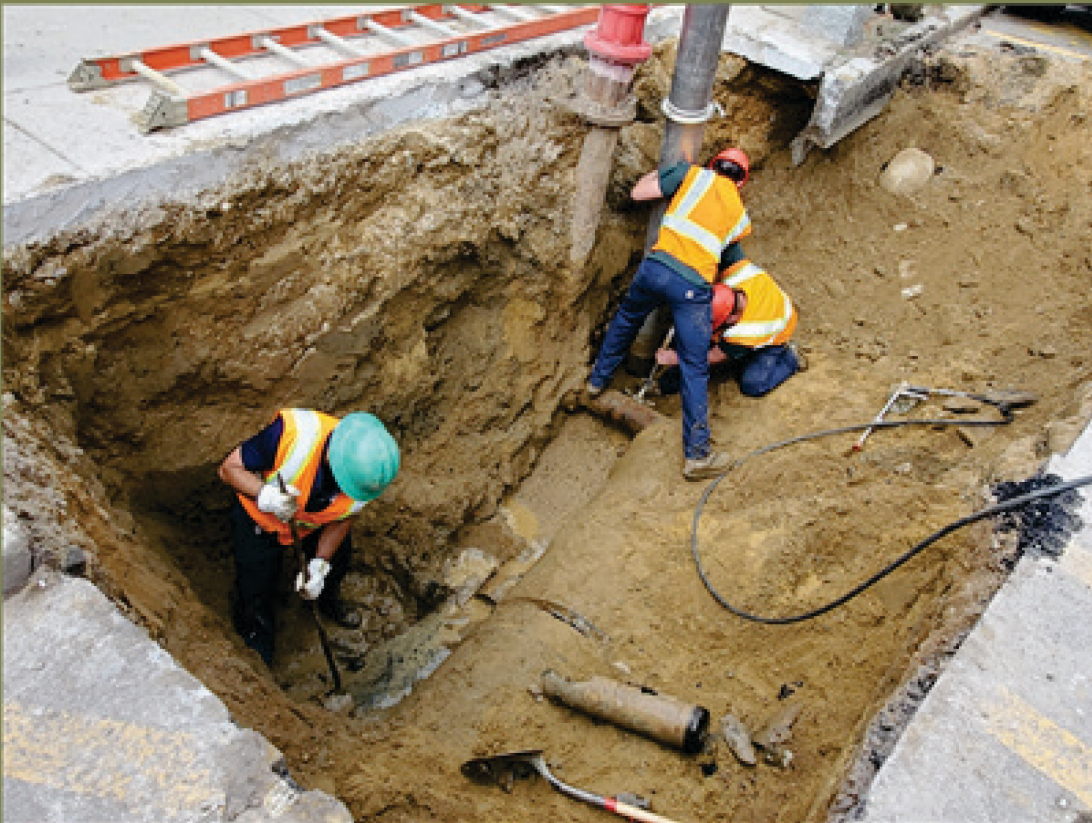
City of Dover Utilities Division working on a project downtown.
