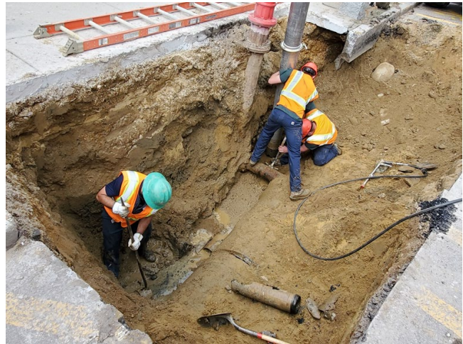
Sewer Service Repair
