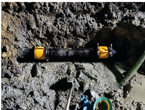
Oak Street repair.
