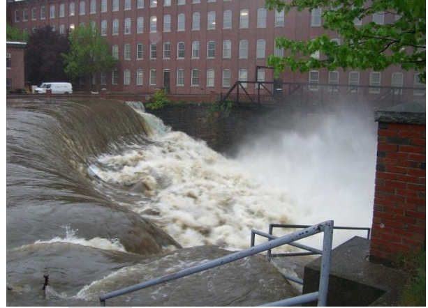
Figure 2: Cocheco River Dam, 2006
