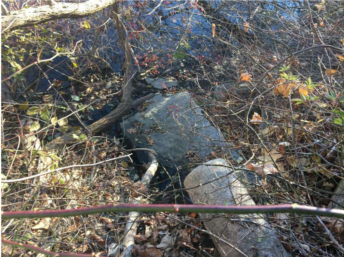
Area of impact, existing culvert outfall
