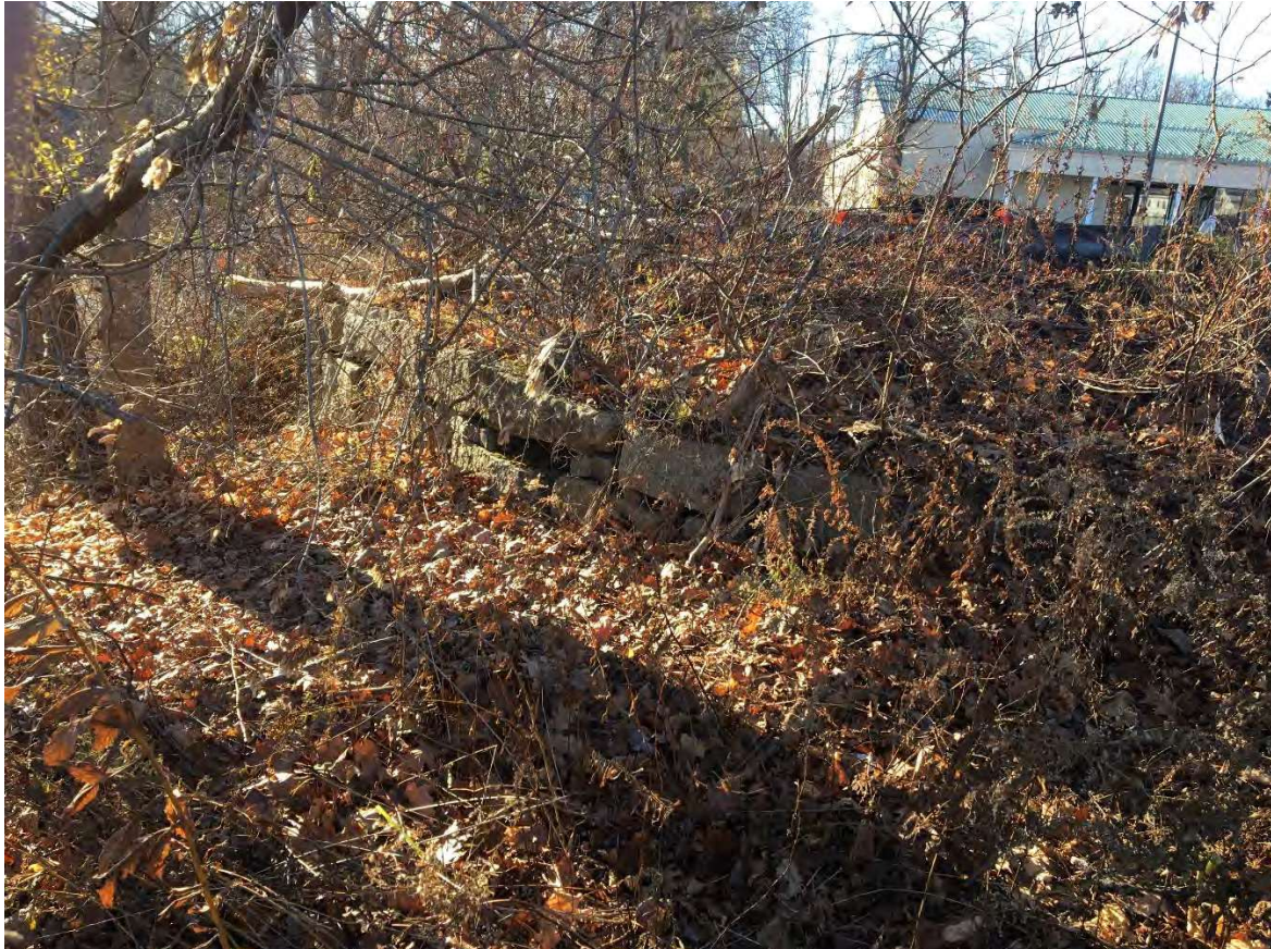
Existing retaining wall near top of bank, resource is to the left
