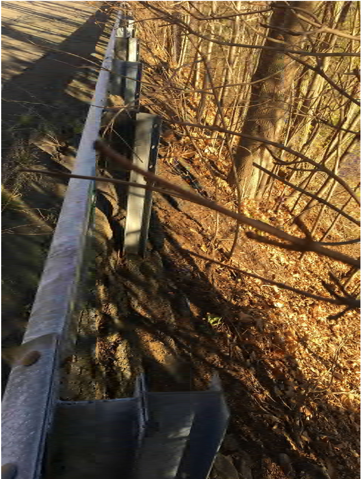
Guardrail at top of bank, resource is to the right
