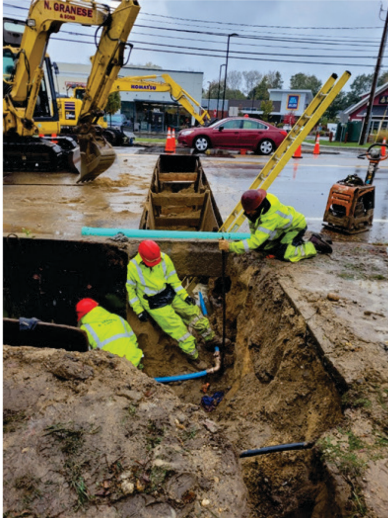
New 2" water service for THE HERBAL PATH
