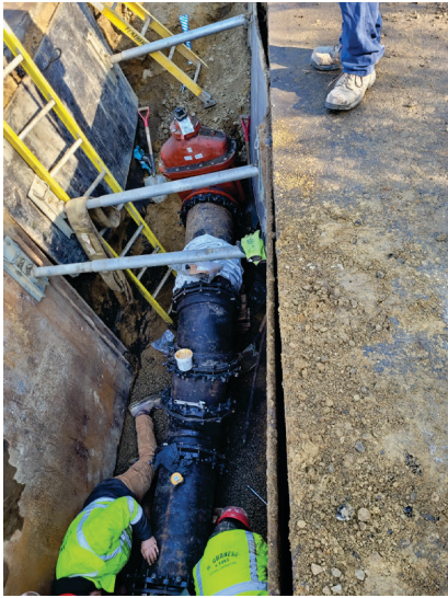
Lowell Ave water main tie in.
