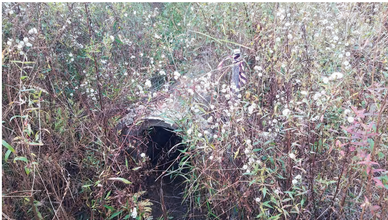
Photo 5 – Culvert under Route 9 with connectivity to Wetland A. (Photo taken 10/21/21).
