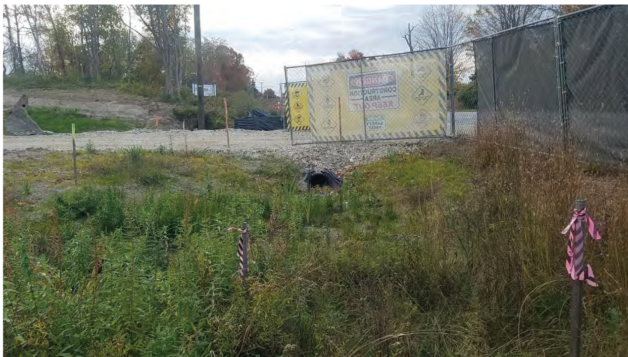
Photo 6 – Culvert under site driveway with connectivity to Wetland A. (Photo taken 10/21/21).
