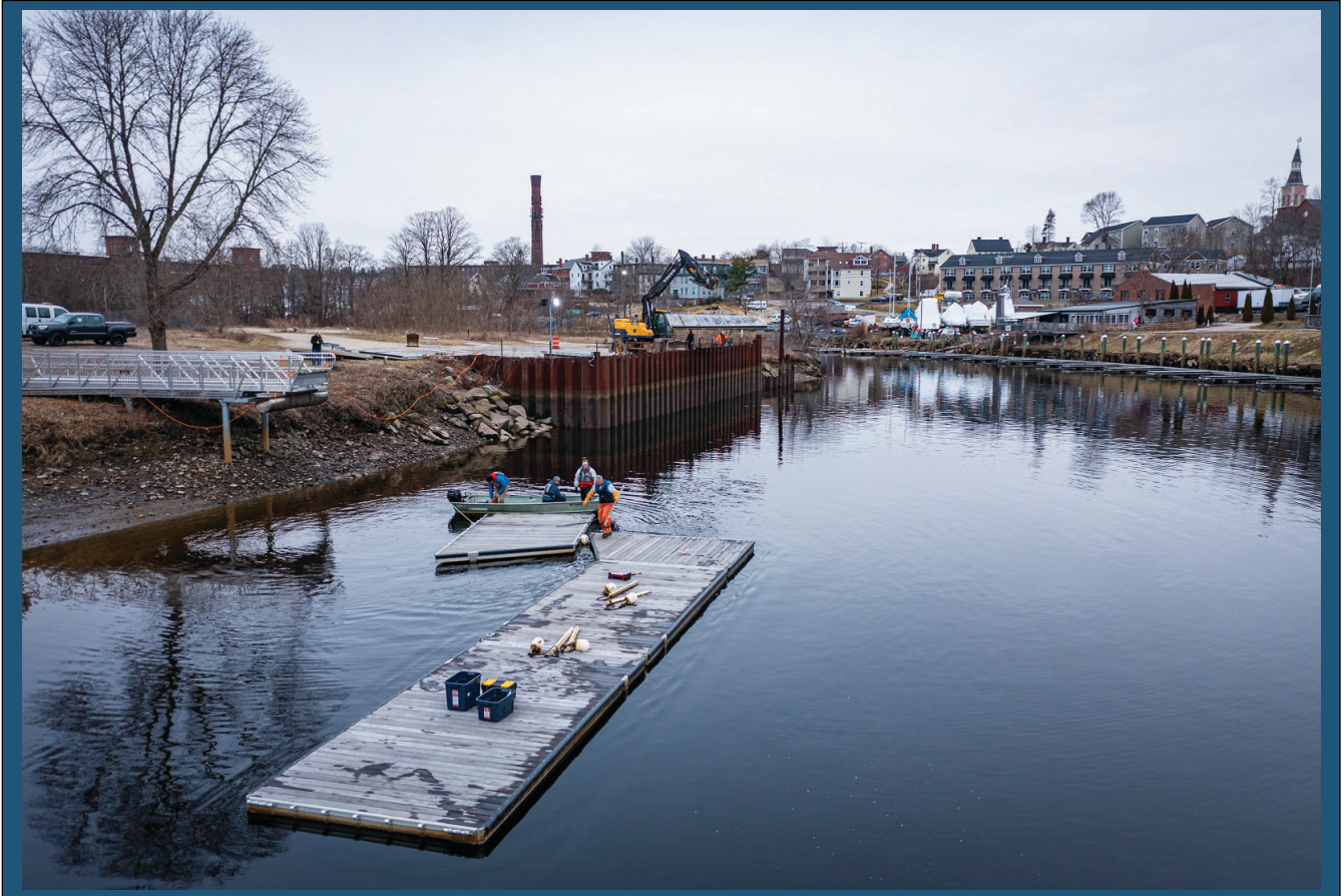
Seasonal installation of the Paddlesports Dock on the Cocheco River, 2022
