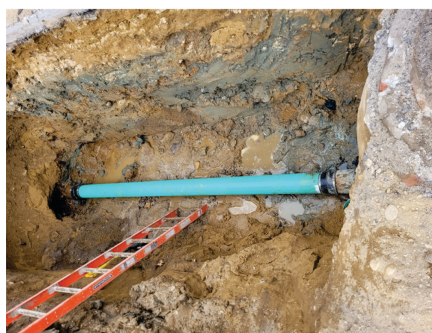
Sewer Main repair Hampshire Circle
