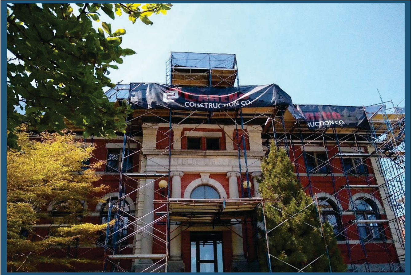
Public Library Roof Replacement Project, May 2022
