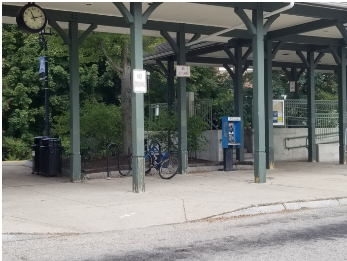
View of access from parking
