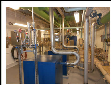
Four new Aerzen Channel and Septage Blowers and Two new Carter Plunger Pumps
