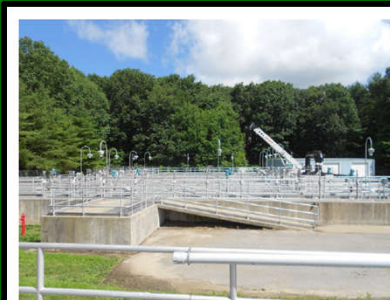
MLE Process with Invent Mixers and Aquarius Technologies Aeration System
