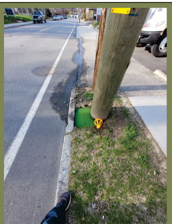
Dye tested sewer service to confirm hit lateral.
