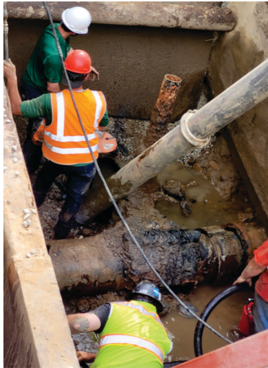
Exposing the water main.
