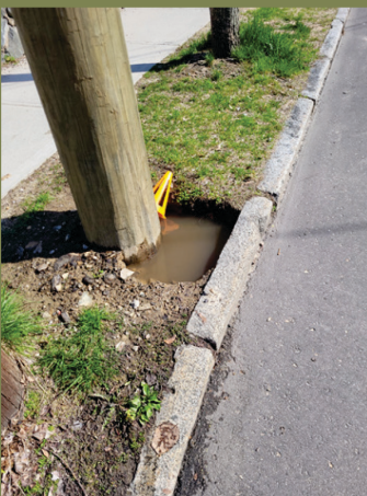
Reported water around telephone pole.
