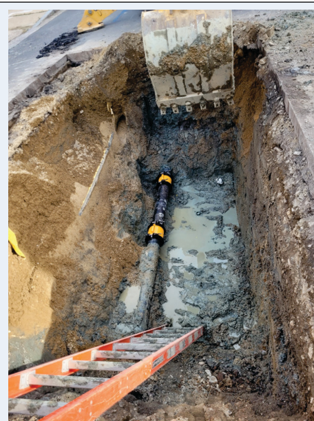
Repair to cast iron water main, Atkinson Street
