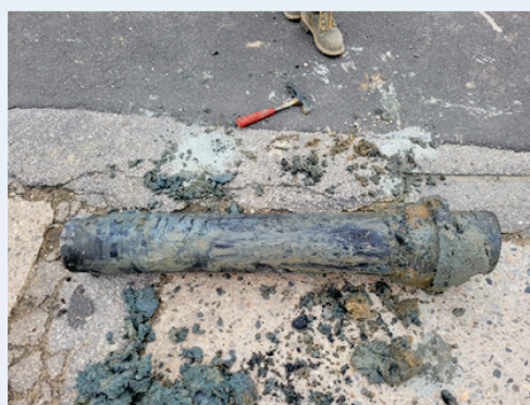
Cast iron water main, Atkinson Street
