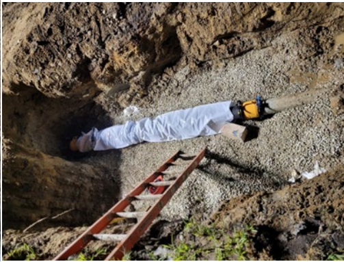
Tanglewood Water Main Post-Repair
