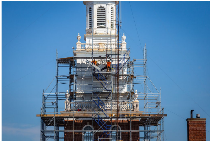
City Hall Clock Tower Remodel
