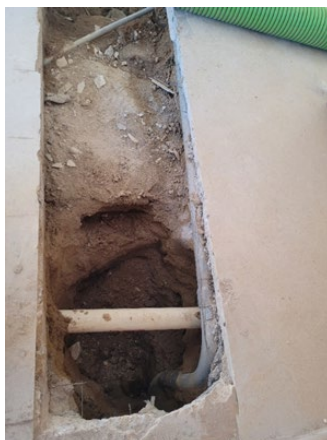
City Hall floor for elevator repair.
