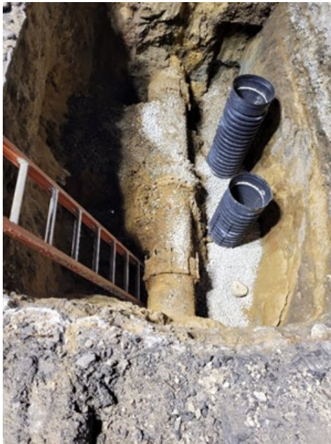
Central Ave Gate CI Water Main
