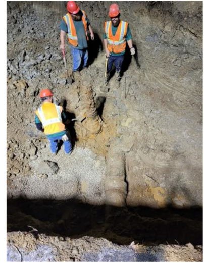
Crosby Road, Water Main
