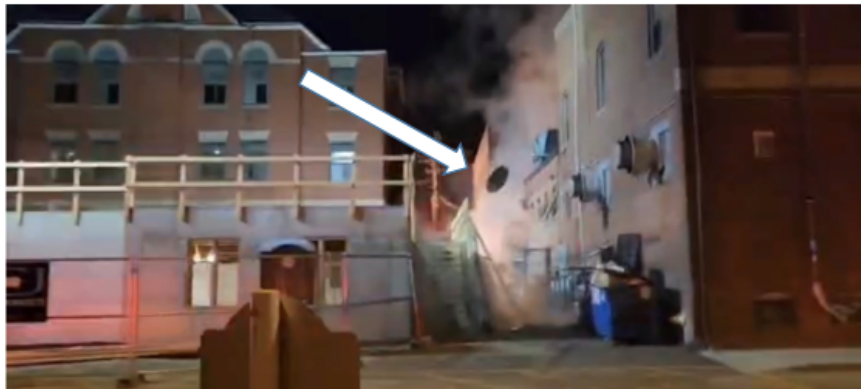
Photograph from First St. of the lower man-hole just after one of the explosions. Note the 1 lb. cast iron man-hole cover returning from orbit.
