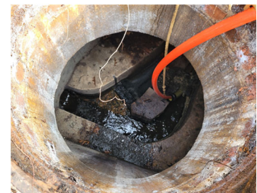
Siphon being cleaned
