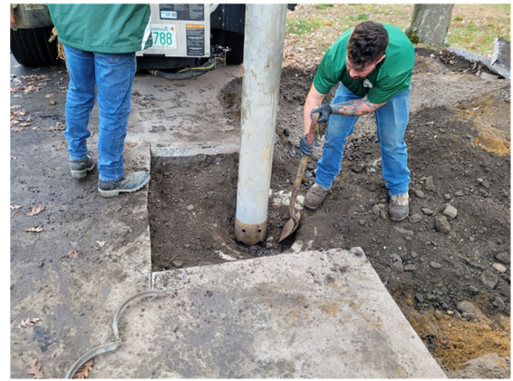
Crew working to clear a sewer manhole in Rollinsford
