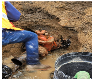
Crews working on removing old valve 56 Sixth St
