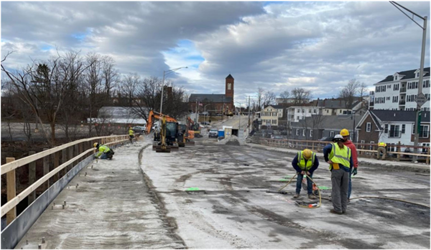
Work begins on the Chestnut Street bridge.
