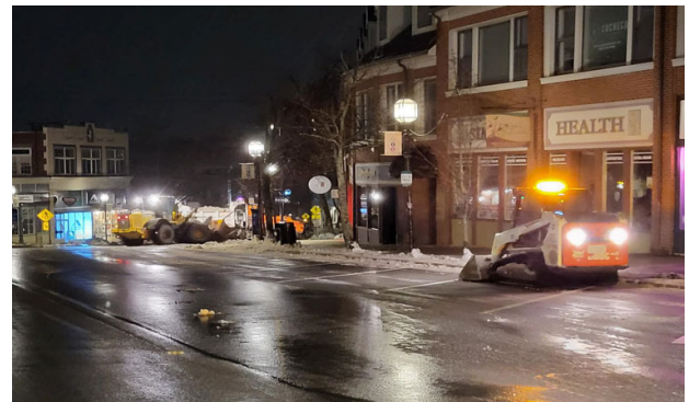
Skidsteer & loader working as a team to cleanup the downtown area.
