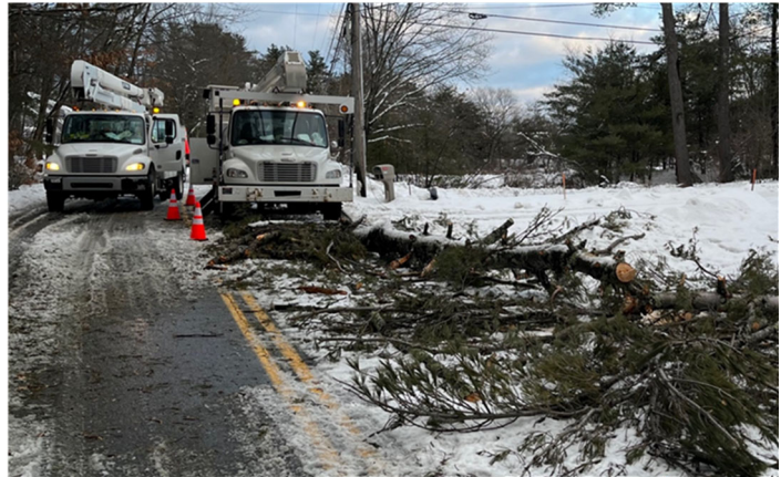
Crews work to restore power at the scene of one of many downed trees during the recent winter storm.
