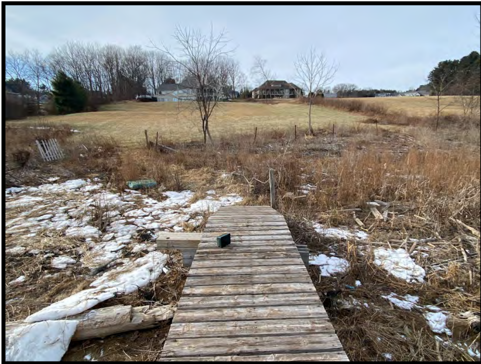
Photo 2. Start of the landward section of dock – to be replaced – Facing south
