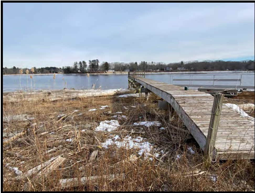
Photo 1. Existing Dock – 50' section to be replaced (section w/out railings) – Facing north
