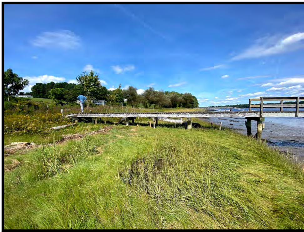
Photo 6. Existing dock – section to be replaced (up to railing) – facing west
