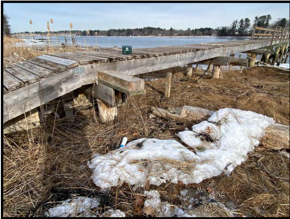
Photo 3. Section of Dock to be replaced (up to railing) – Facing northeast
