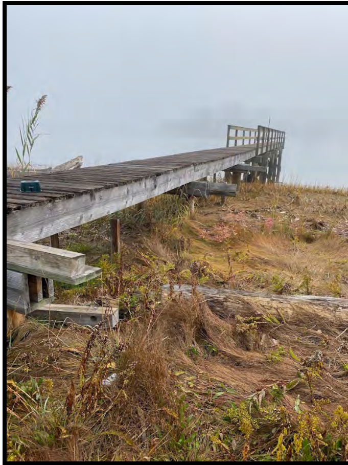
Photo 5. Existing dock – section to be replaced (up to railing) – Facing Northeast
