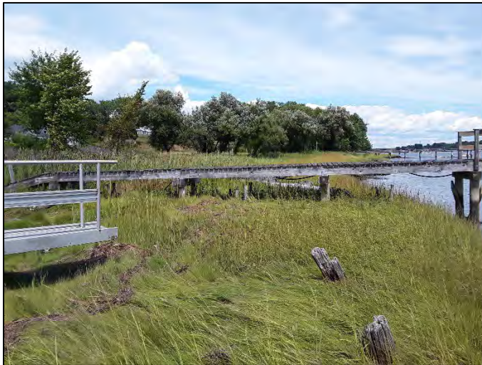
Figure 3: Saltmarsh area around dock structure
