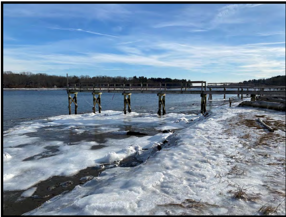
Photo 4. Existing Dock – side profile. Facing East
