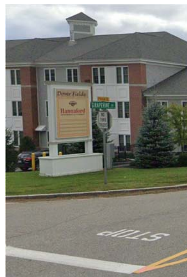
Existing secondary entrance at Mast Road (Courtesy of Google Streetview ©2023)
