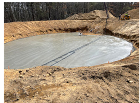
Foundation prep for the new water storage tank on Smith Well Rd.
