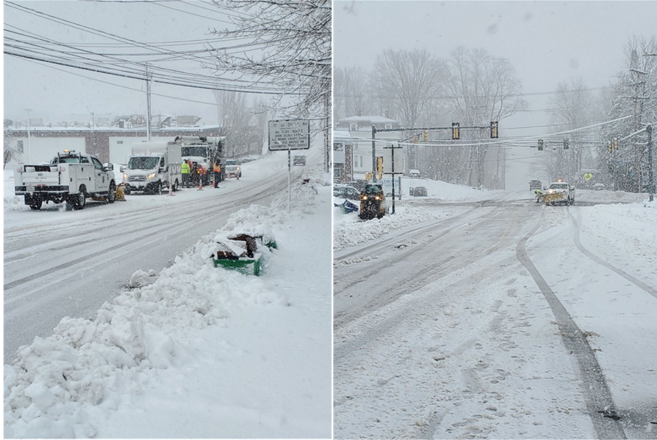
Utilities & Streets Crew working to clean the line.
