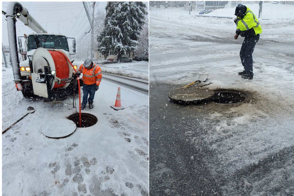
Above left: Utilities foreman working on opening the sewer manhole at Oak St and Broadway. Above right: Utilities foreman verifying that the sewer jet is passing through the manhole.
