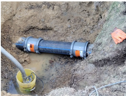
Above: Repair on Constitution Way
