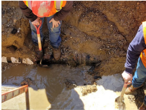
Above: Crews working on Hough St leak
