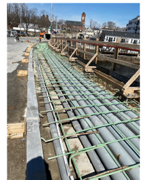
Eastern sidewalk on Chestnut St Bridge with new utility conduit and reinforcing. Sidewalk concrete being poured in the background.
