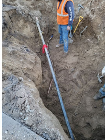
Above: Grove St renewed service line
