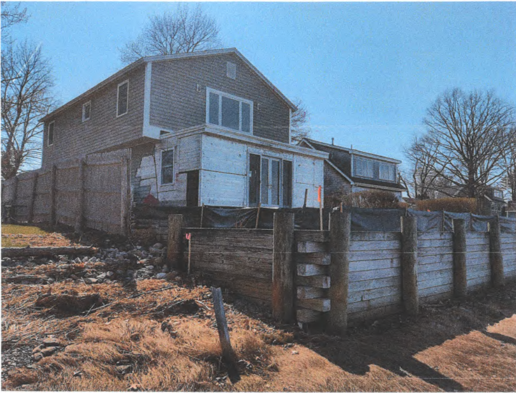
5. Looking west at the house and the eastern corner of the retaining wall.
