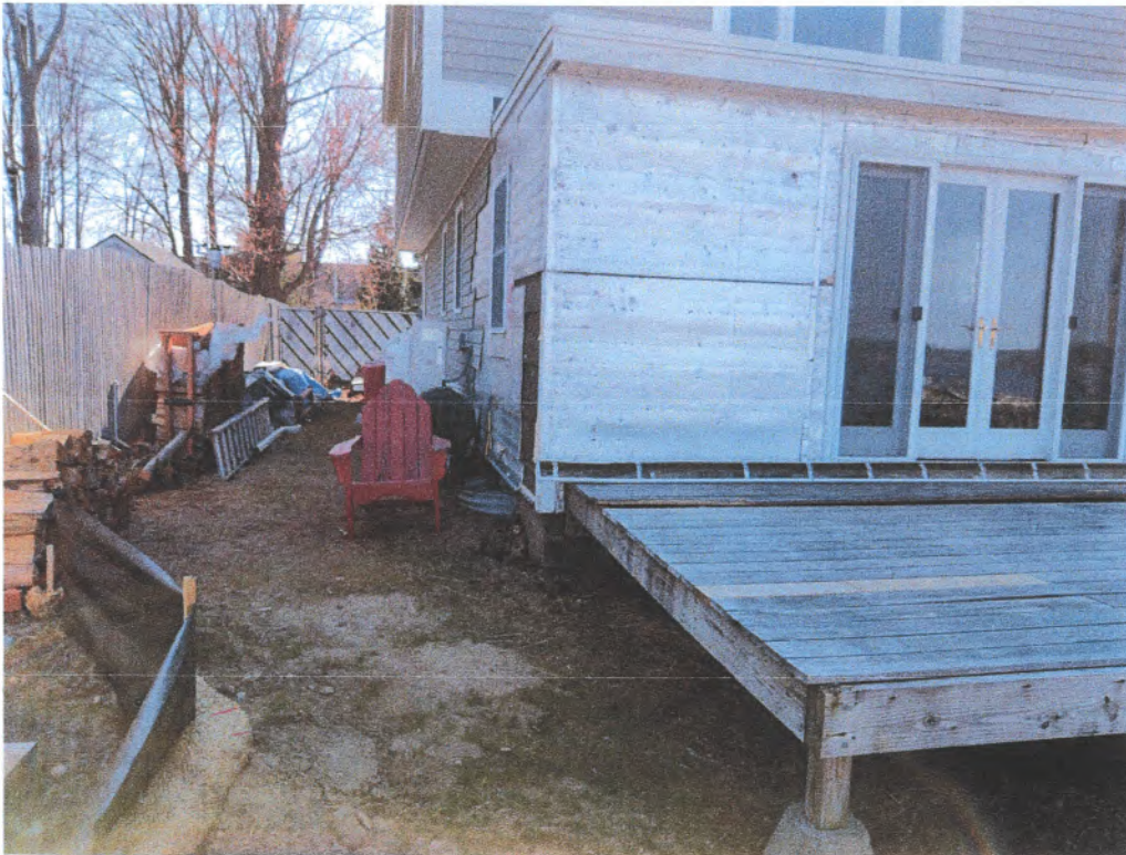
6. Looking southwest at the temporary impact areas south of the house.
