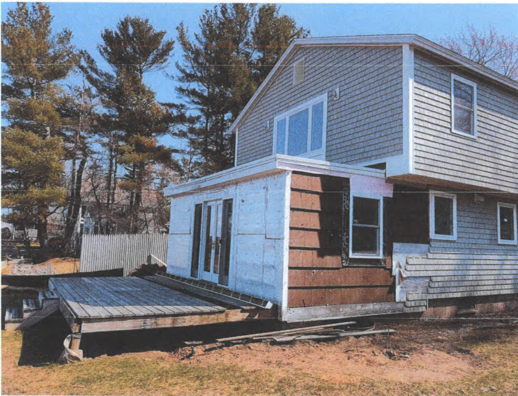
2. Looking southeast at the deck to be replaced and the room where the 2 nd story will be added.
