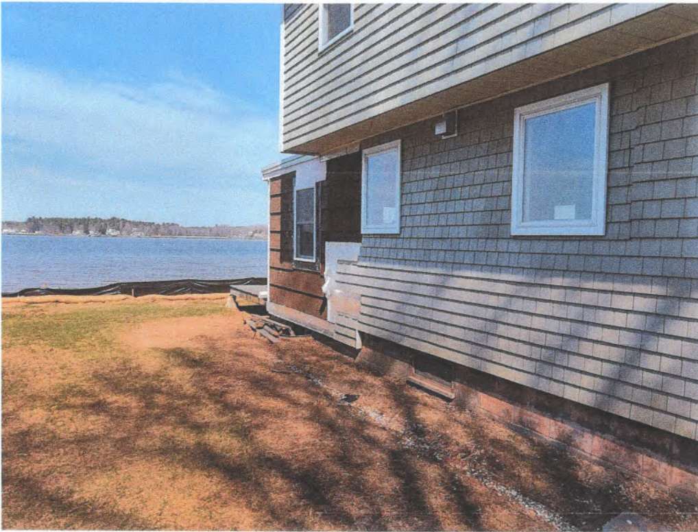
1. Looking northeast at the temporary impact area.
