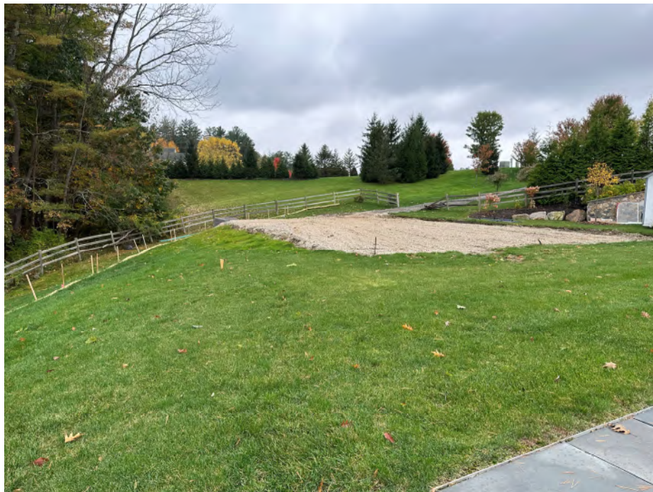
Photo #2: Looking southerly at area roughed out for proposed sport court. – October 17, 2022
