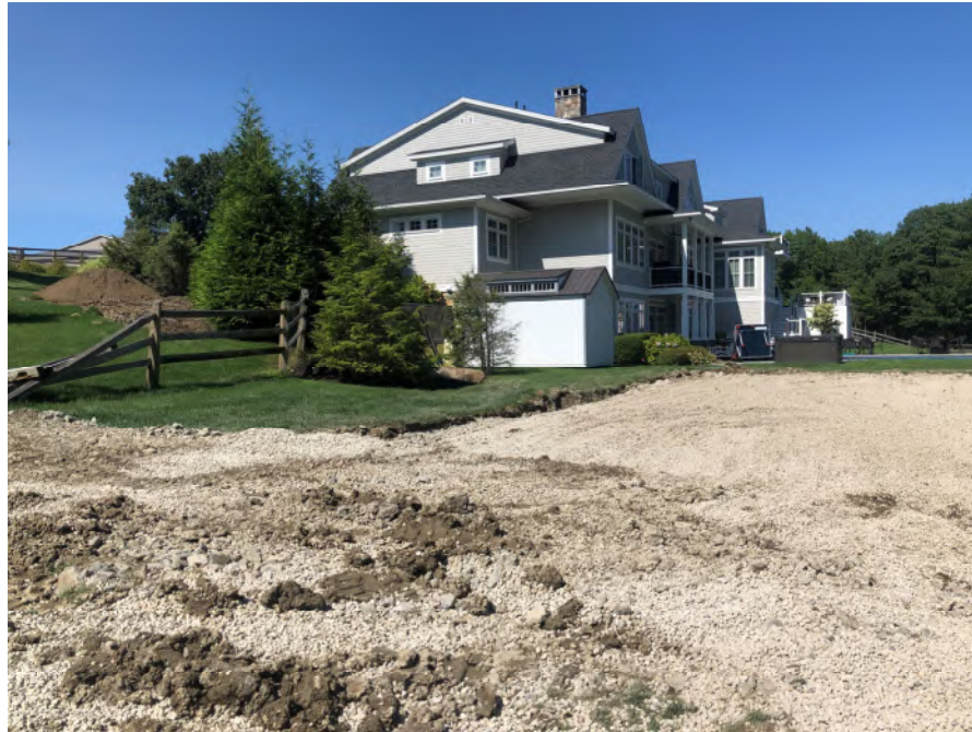
Photo #5: Looking northerly at existing residence. Sport court to be constructed in previous lawn area. - September 8, 2022
