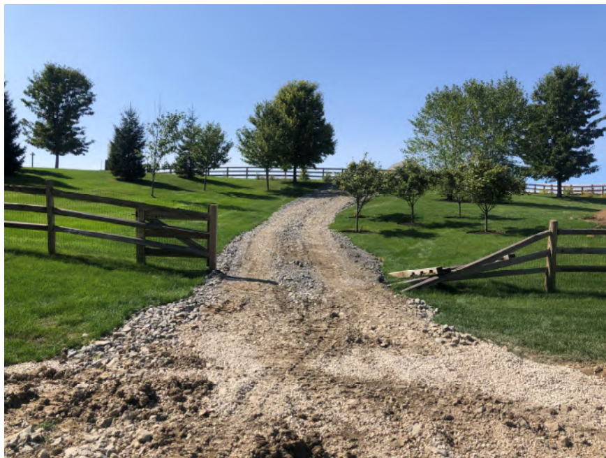
Photo #4: Looking westerly at existing temporary access drive installed for the construction and future access to sport court and pool area. September 8, 2022
