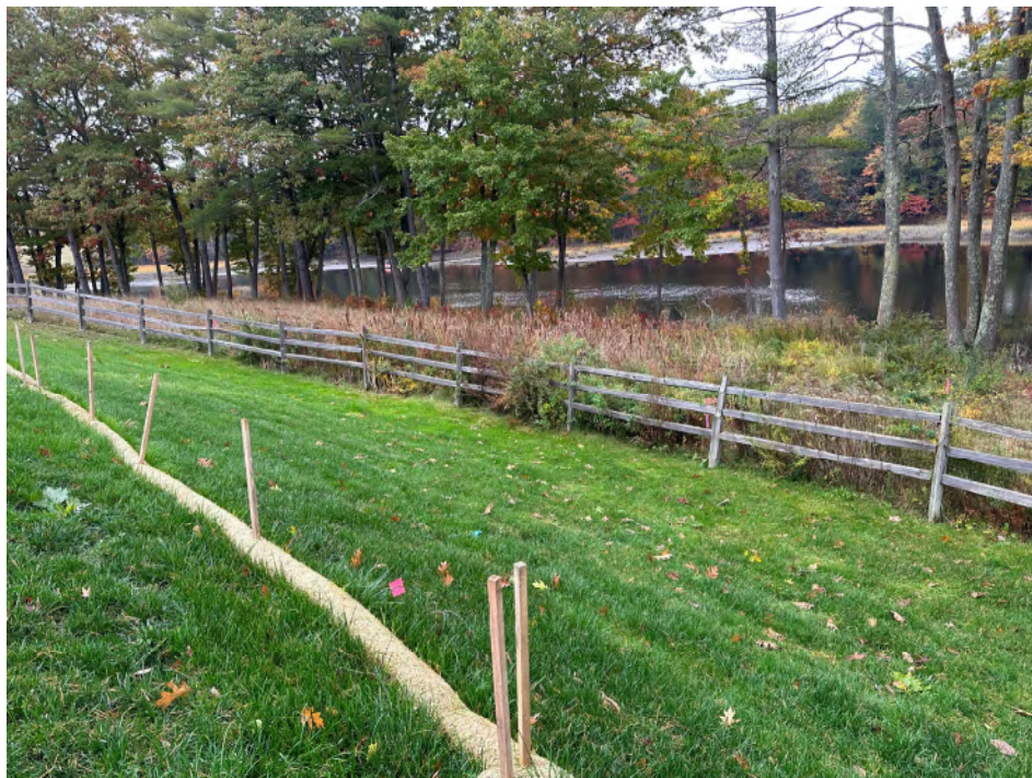
Photo #6: Looking easterly at existing sediment tubular barrier, lawn, fence and waterfront trees and river beyond. October 17, 2022
