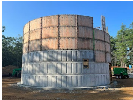
June: Pedestal for Smith Well Road Elevated Tank
