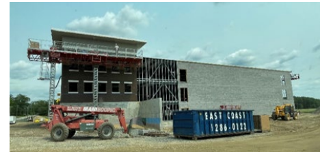
Brick installation on the future Bluebird Storage on Littleworth Road.
