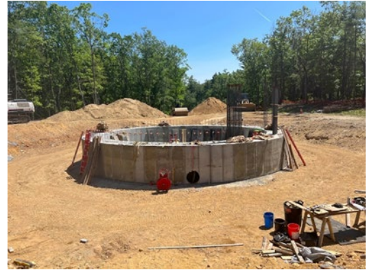
Foundation Ring Wall for Smith Well Road Elevated Tank
