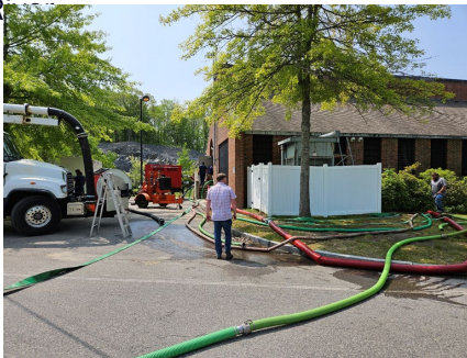
Crews installing pumps.
