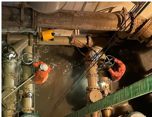
Crews isolating the leak.
