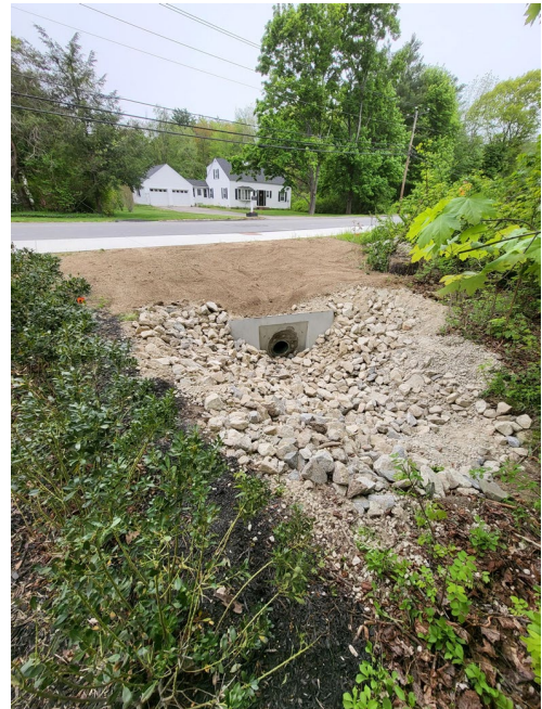
Whittier Street Headwall
