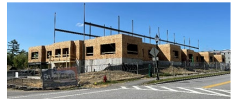
Sitework at residential project at 757 Central Ave.
