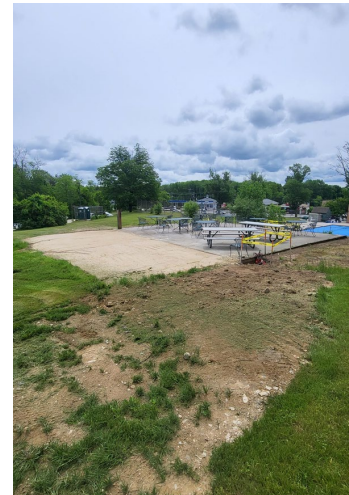
Outdoor pool after pavilion was taken down and cleaned up
