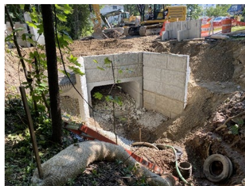
Installation of new precast concrete box culvert below Hough Street.
