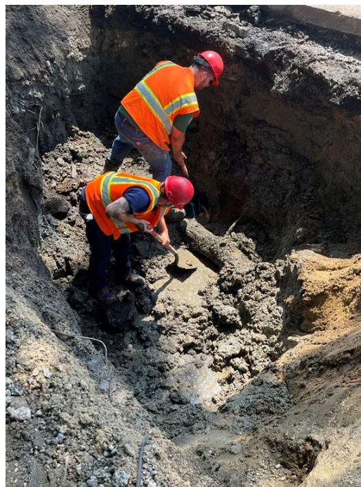
Oak Street water main repair.
