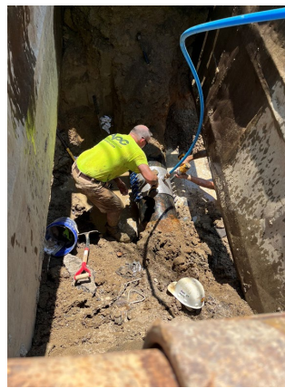
Court Street water service repair.
