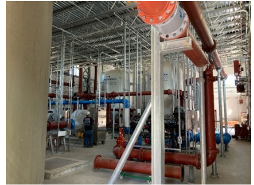
Interior fit up at the new Pudding Hill Water Treatment Plant.
