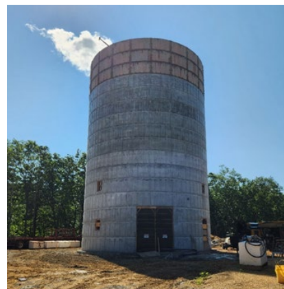
New elevated tank pedestal continues to rise.
