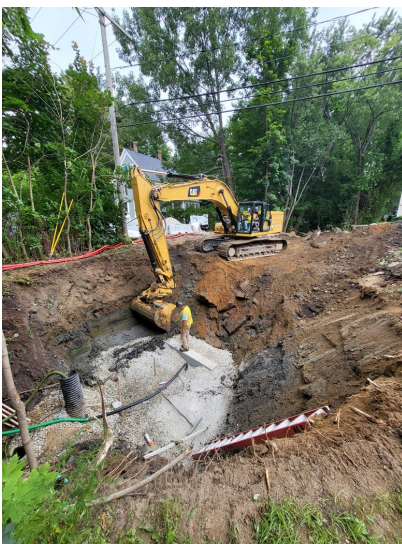
Hough St project. SUR digging for and starting to set the outfall headwall pieces.
