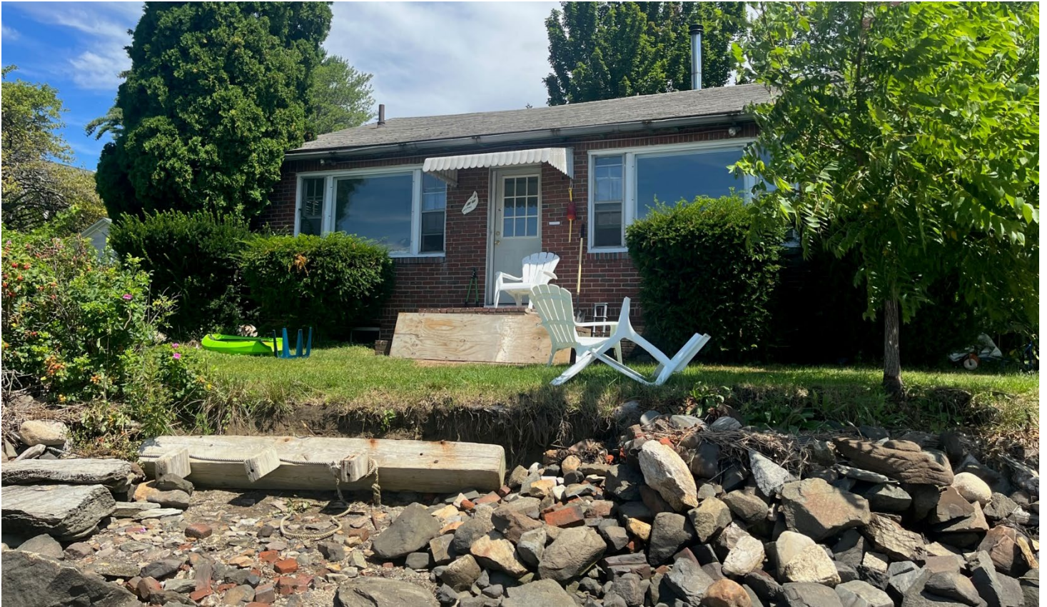
Photo #11: Looking northeast at existing residential dwelling from shoreline.
