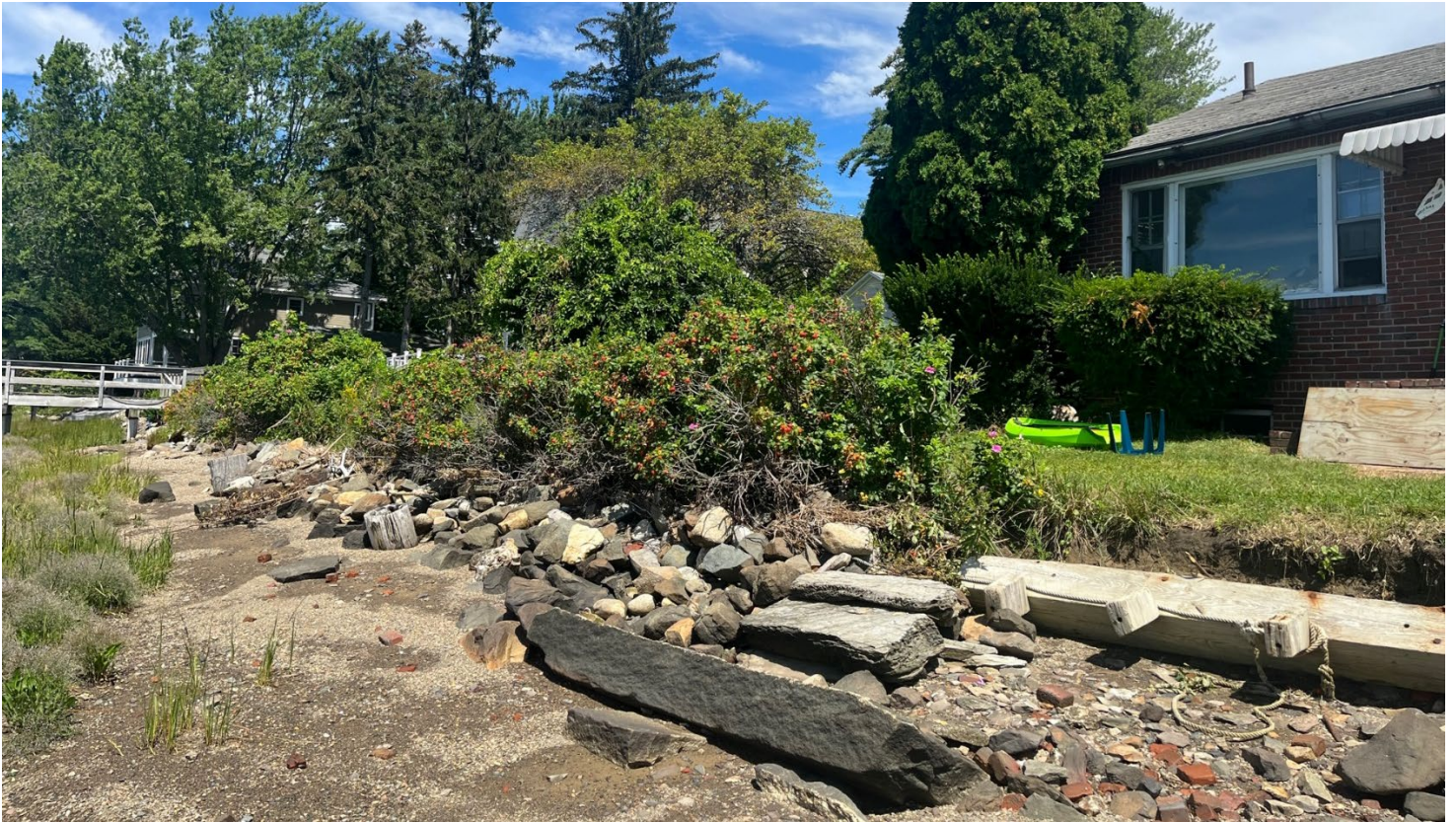
Photo #13: Looking northwest at existing residential dwelling adjacent to shoreline.
