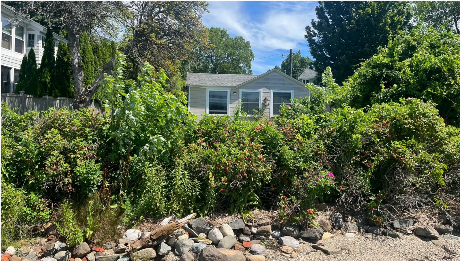
Photo #15: Looking northeast at existing residential cottage.
