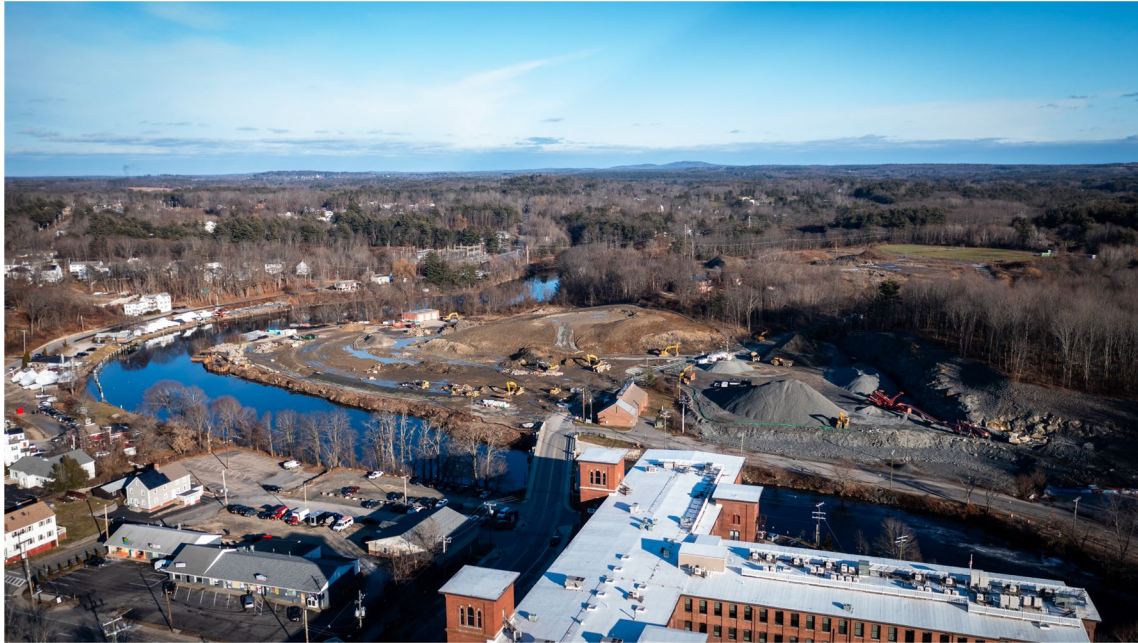
A view of the current progress on Waterfront.
