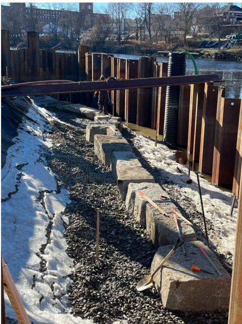
Granite being used to build shoreline stabilizing wall.
