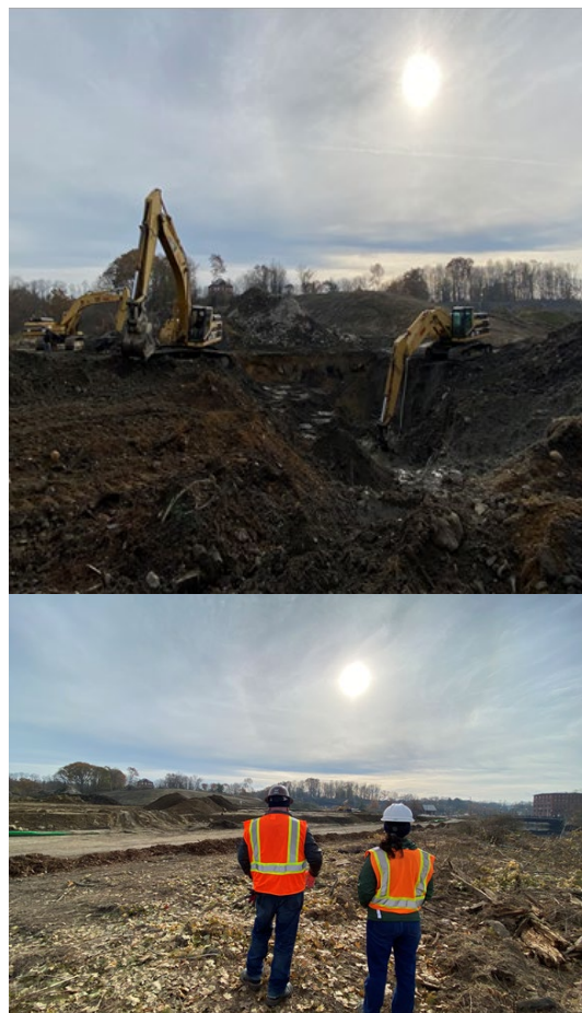
Excavation of the former WWTP Clarifiers (top). Waterfront Construction Manager Jamie Stevens and Assistant City Engineer Jillian Semprini, PE oversee work on the Waterfront.
