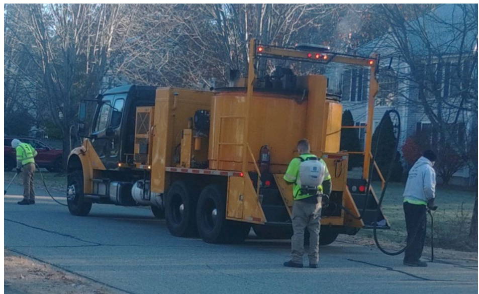
Indus industries crack sealing in the Alden woods neighborhood
