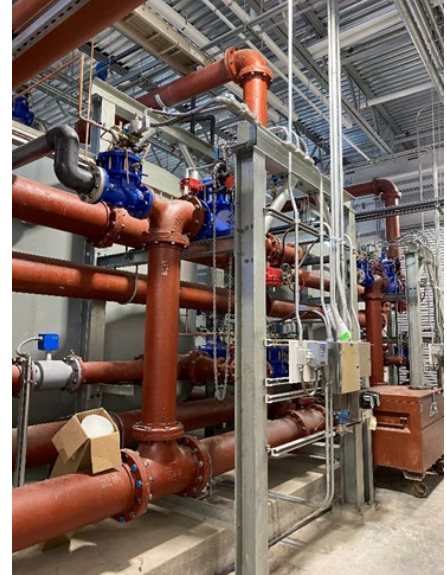
Work continues on the Pudding Hill Treatment Plant.
