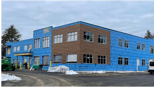
7 West Durham Road Medical Office
