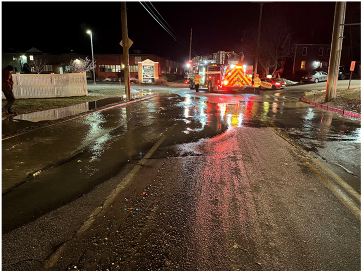
Water Main Break Locust Street
