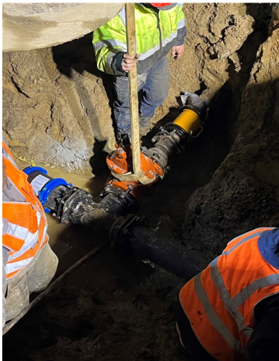
New Valve Installed High Ridge Drive
