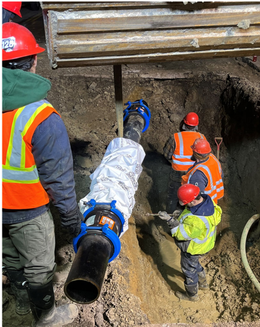
Installing repaired section of water main on Locust Street.
