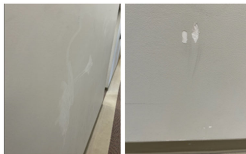
Administration hallway walls
