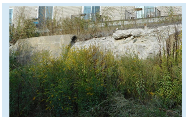
Existing retaining wall
