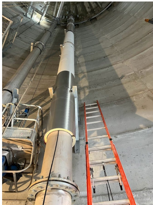
Interior fit up of the new elevated storage tank near Exit 9.
