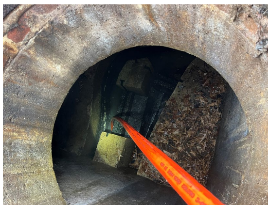
Cleaning the siphon
