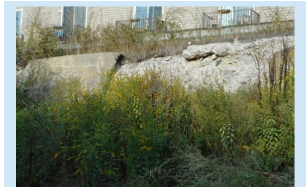
Existing retaining wall
