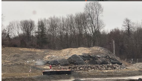
Sitework and blasting continues on the waterfront.
