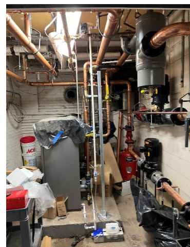
Library Boiler at approx. 75% complete.
