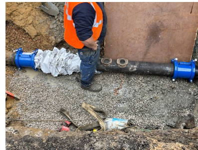
Oak Street repair
