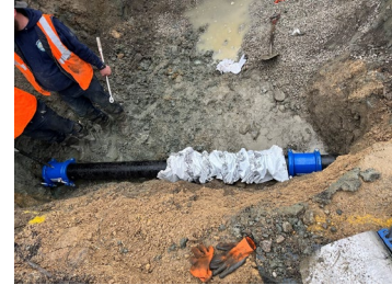
Rollins Road repair
