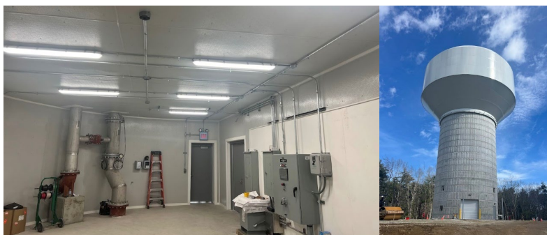
Interior of the new elevated storage tank pedestal and exterior view of the tank nearing completion.
