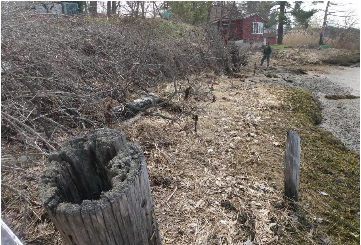
Photo 2 Bank wave erosion. By CNE on 4-11-23
