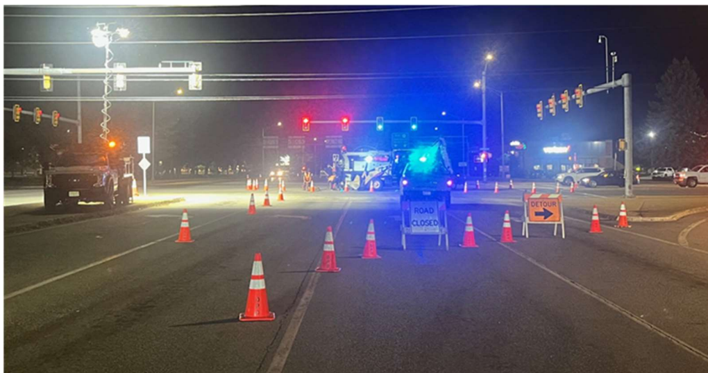
Crews work to repair a sunken sewer cover at Weeks Crossing.
