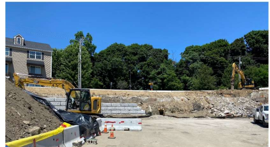
Portland Avenue Retaining Wall is rising.
