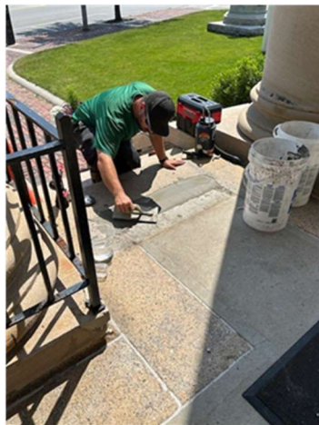
City Hall front step repair
