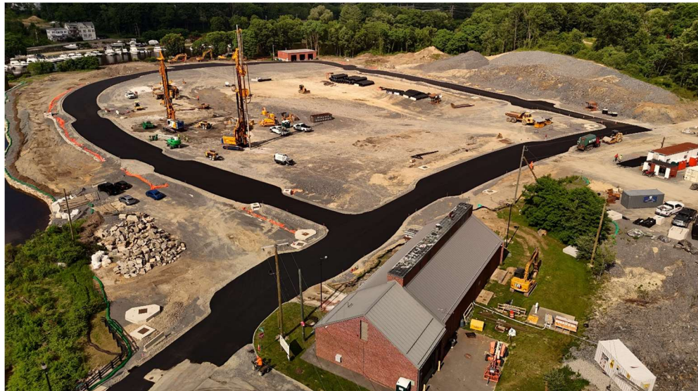
Base course pavement has been installed at the waterfront redevelopment site.
