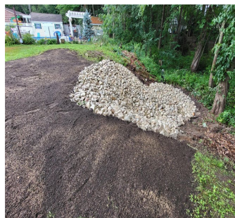
Crew repaired outfall on Oakhill Drive.
