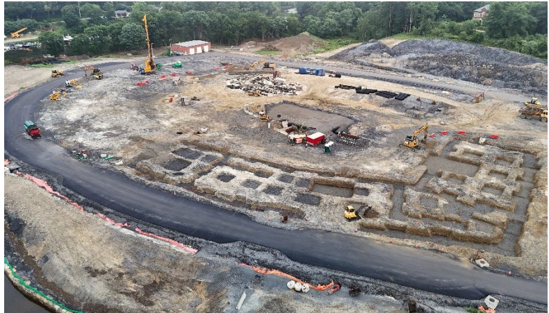
Waterfront foundation progress on building C.
