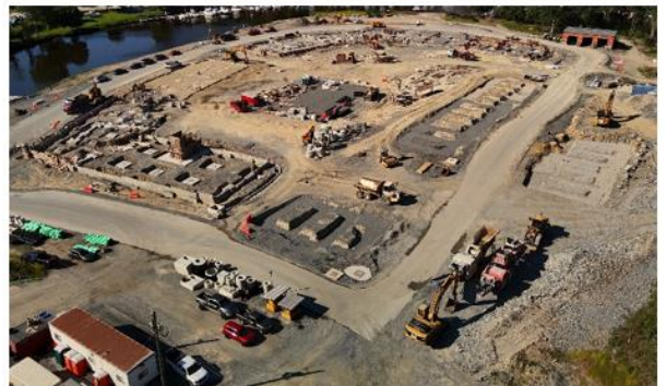
Foundation work for the private development continues to prepare for vertical construction.
