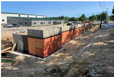
Inspection Services' new building foundation is
