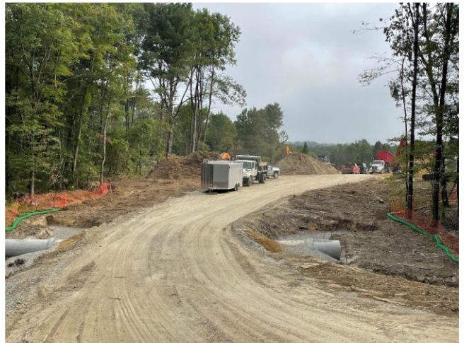
59 Tolend Rd Residential Housing project kicked off in August.
