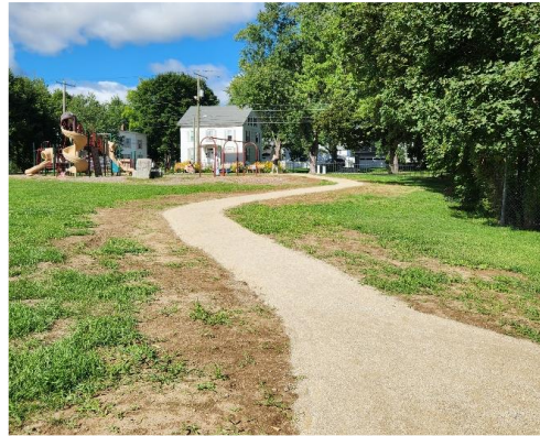
New Pathways at Park Street Park.
