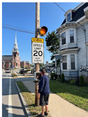
Testing School Zone Traffic Lights
