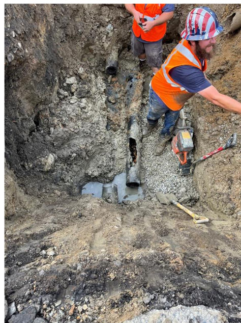
Water Street water main repair.
