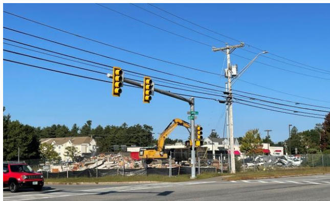
Demolition of the R&W Building on Central Ave to prepare for the new Chase Bank.
