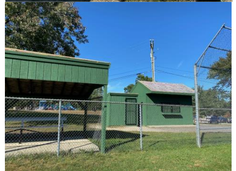
Horne Street School dugout and facility repairs are underway.
