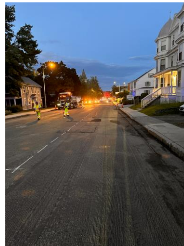
Brox laying out Washington Street ahead of paver.
