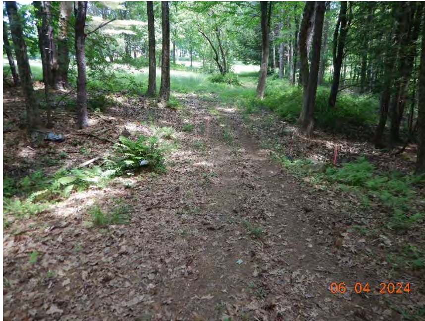
Photo 1 – STA 11+00 Looking East Toward Existing House and Existing Culvert
