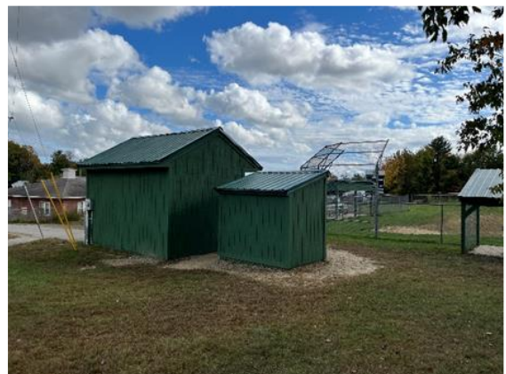
Horne Street baseball field dugouts and facilities received new metal roofs and fresh paint.
