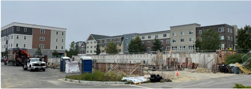
Foundation of 55 Pointe Place is moving along.
