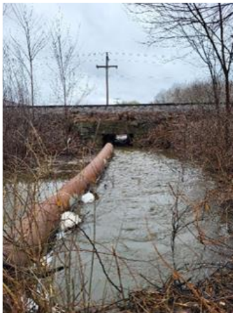
Downstream of the CSX culvert looking back towards Crosby Road.
