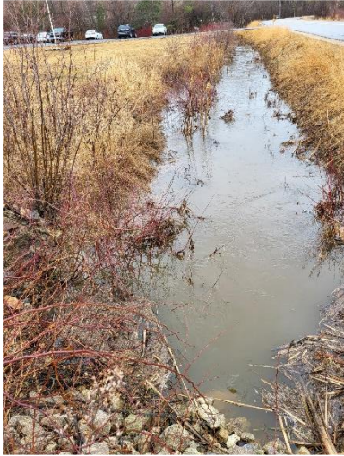
Full drainage channel at Crosby Road.
