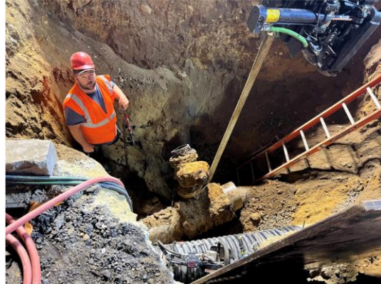
Crews pulling out tee assembly, New Rochester Road
