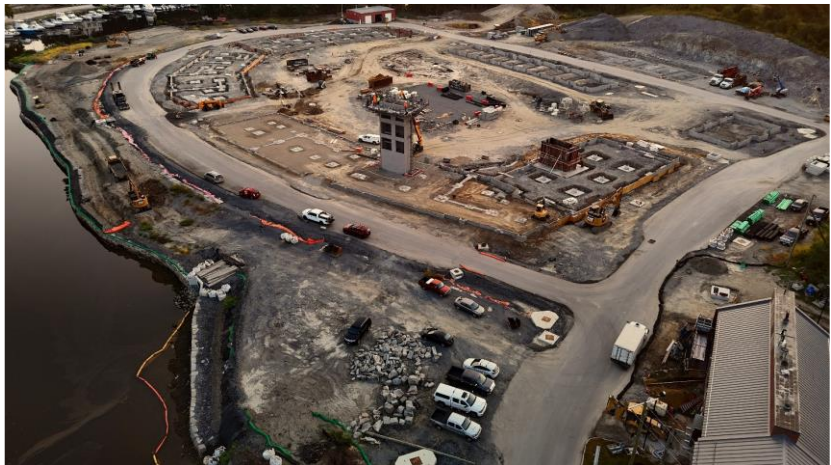
Foundation work on the private development continues with the construction of the elevator shafts.
