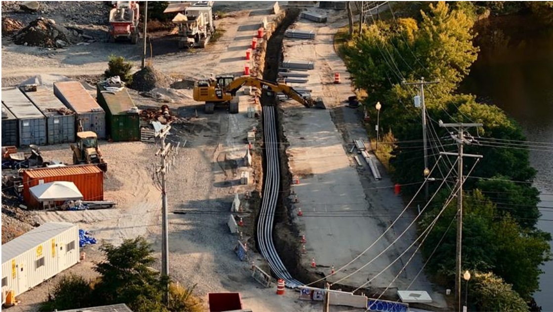
Utility duct bank installation in Payne Street progresses along in preparation for street reconstruction and paving.
