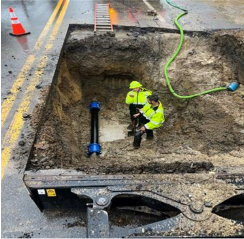
Rainy day Court Street water main repair.
