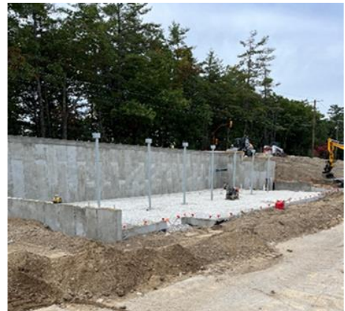
New Inspection Services building foundation is nearly complete.
