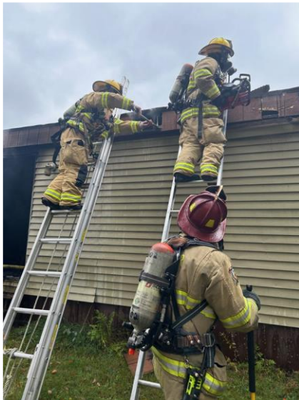
Dover Fire crews working to access fire extension throughout the eaves at Crystal Springs in Somersworth.
