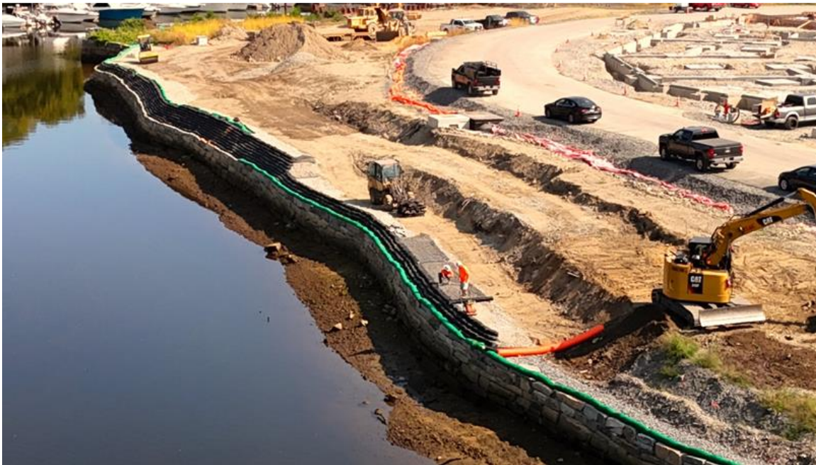
Installation of the flexible mechanically stabilized earth wall (MSE) along the Cochecho River.
