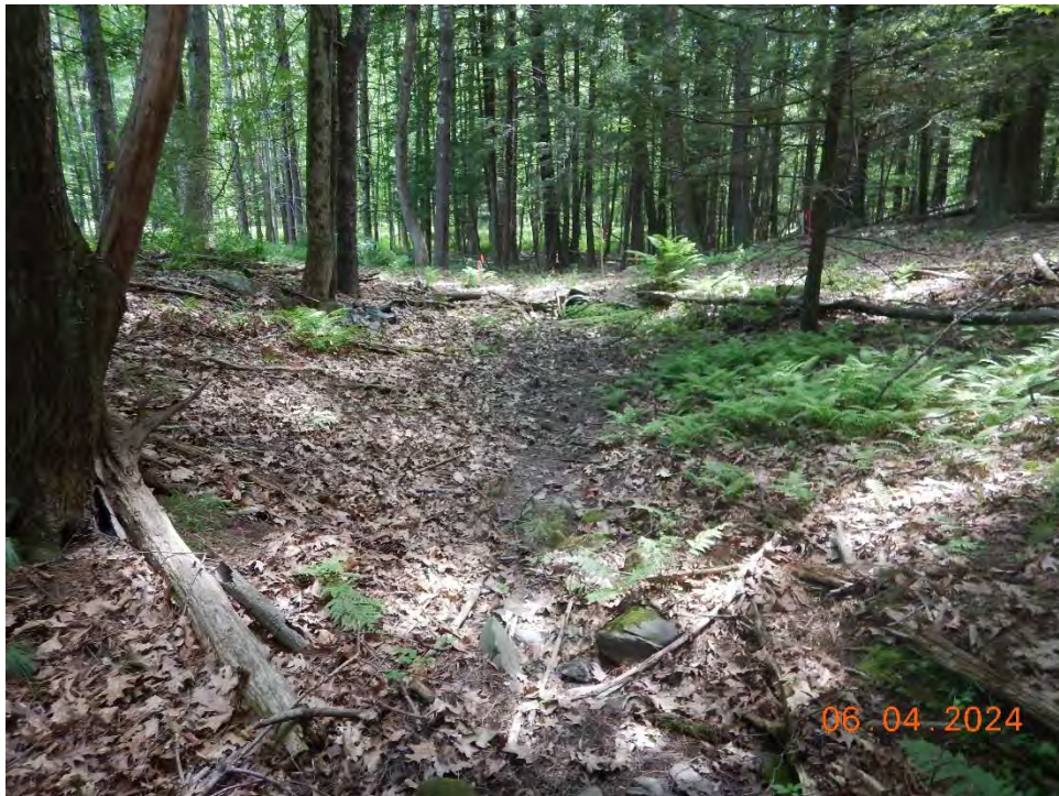
Photo 2 – Inlet Side of Existing Culvert Looking South Toward Woods Road
