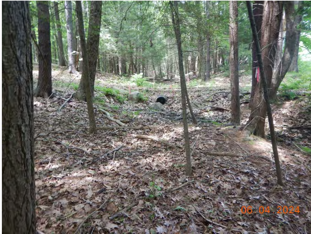
Photo 3 – Outlet Side of Existing Culvert Looking North Toward Woods Road
