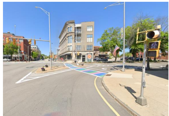
Central Ave and Washington Intersection Signals. The structural components of the signals will be inspected with non-destructive testing methods.
