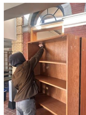
Breaking down library shelving.
