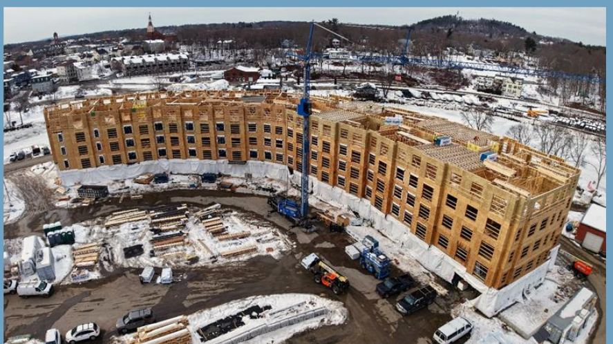
Building D continues to rise high above the Cochecho River.
