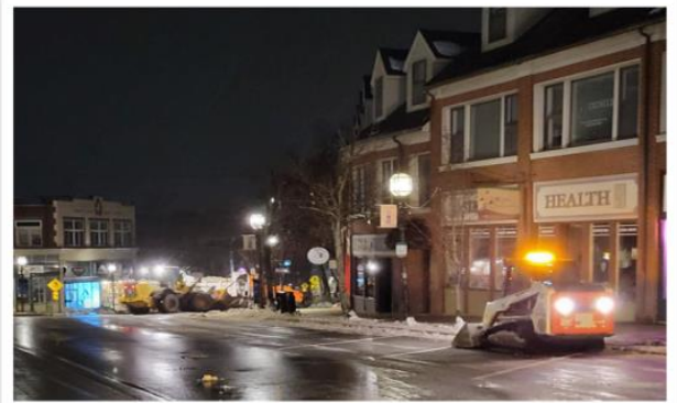
CS crews working in the middle of the night to clear snow from Downtown to restore pedestrian and parking access.
