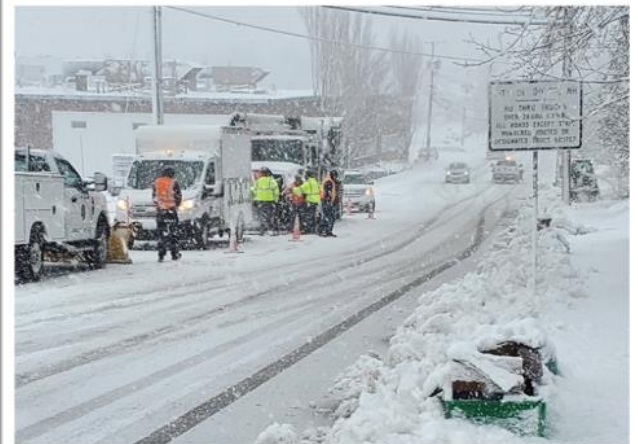
CS crews responding to a sewer main backup during a snow storm while another CS crew member clears snow from the sidewalks.
