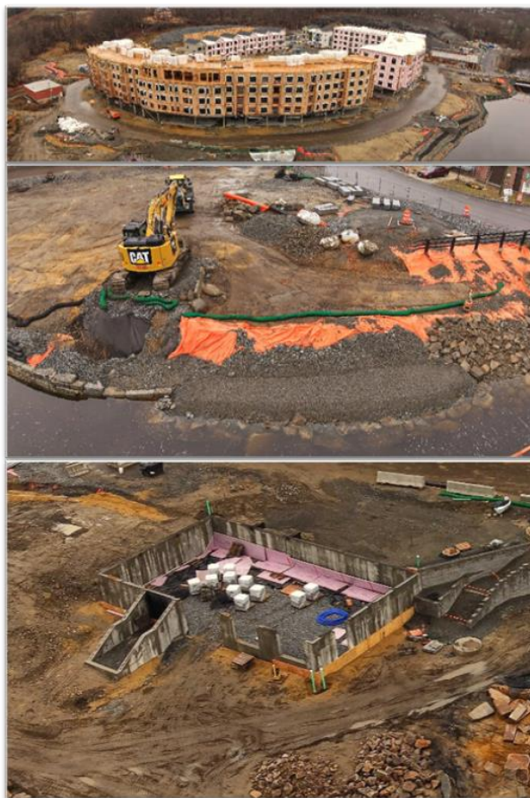
Construction of the Waterfront Pavillion
