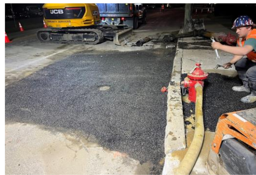
Wrapping up the Central Ave break.
