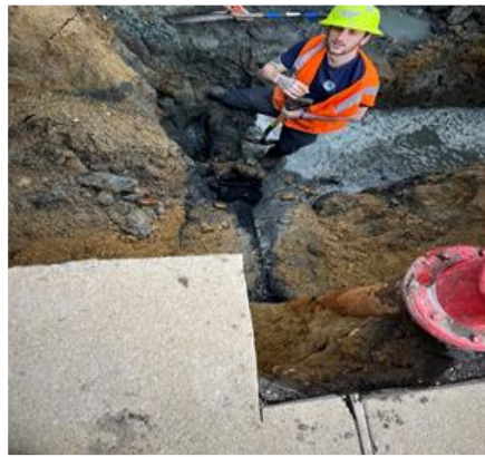
Broken valve replacement
