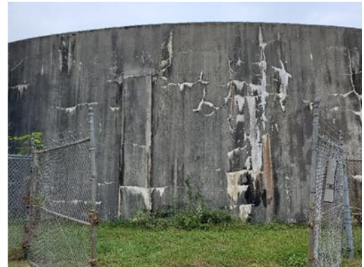
Existing Garrison Hill Tank has been drained and inspected.
