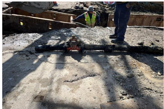
Portion of broken water main removed on Angle St @ Central Ave
