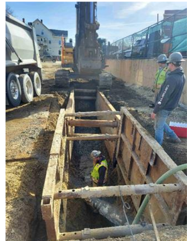
Utility replacement continues on Angle Street
