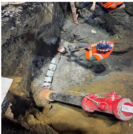
Broken valve replaced with a new hydrant
