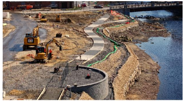
Riverwalk Construction on the Waterfront is moving along.
