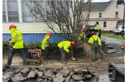
Granese crews rebuilding a retaining wall adjacent to the project as part of the finish work on Grove Street.
