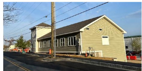
Inspection Services building is almost complete.
