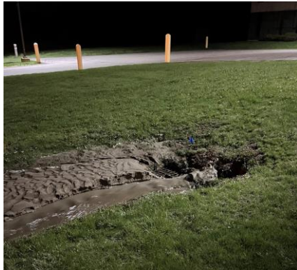
Fire line main break Crosby Rd
