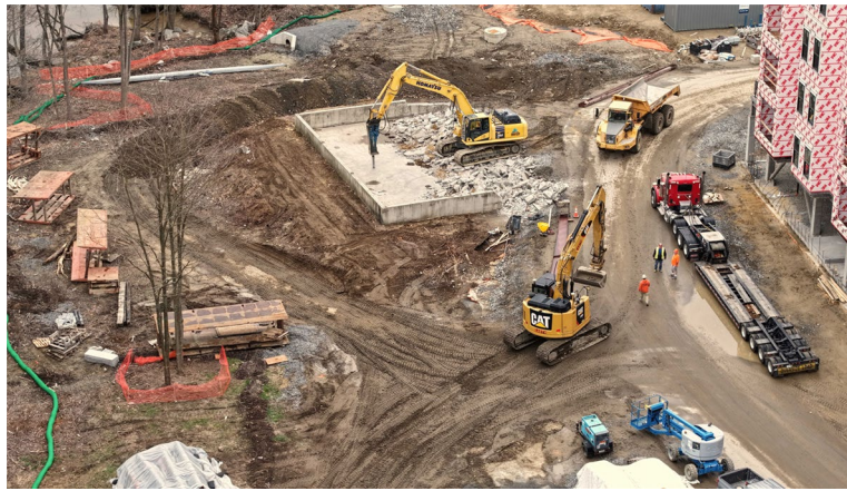
Demo of Maintenance Building
