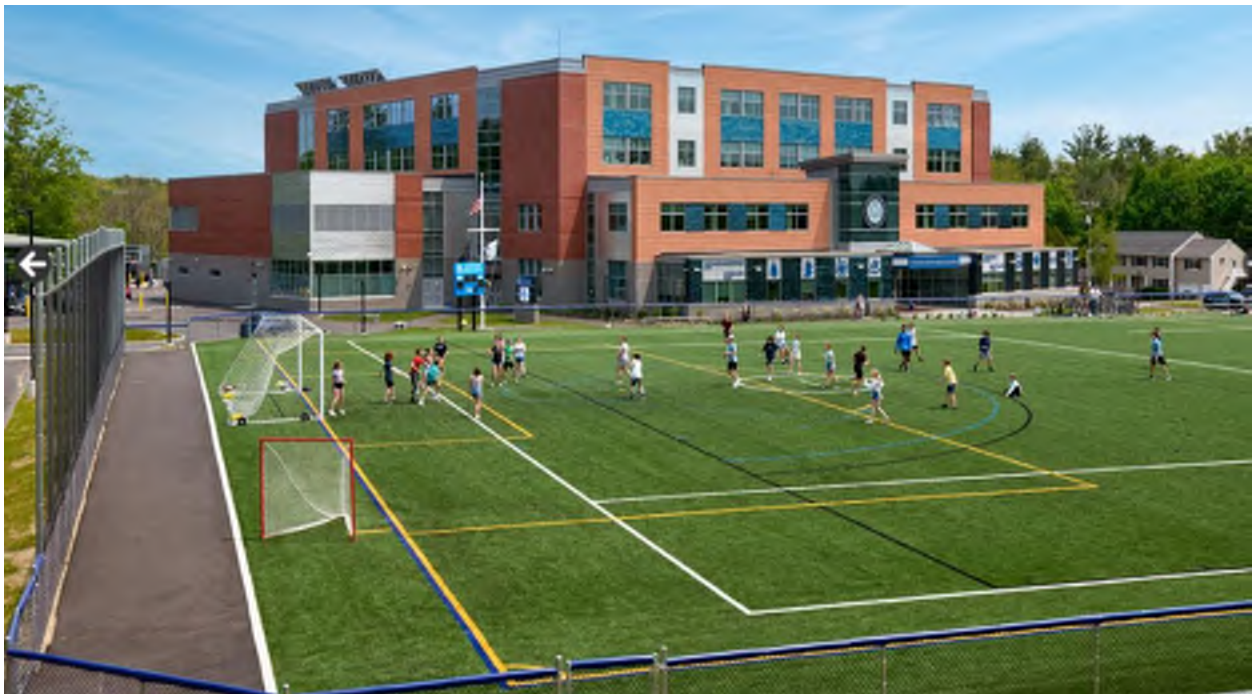
Oyster River liked the synthetic field they built at the high school in 2016 so much, they built a second one at the new middle school that opened in 2022.
