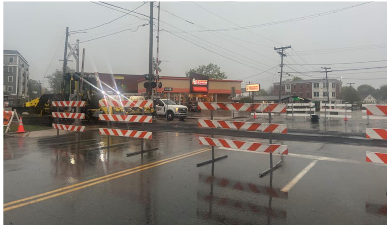
Central Avenue railroad crossing closure on May 2-3, 2025
