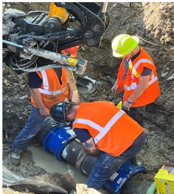
Oak St Water Main Repair
