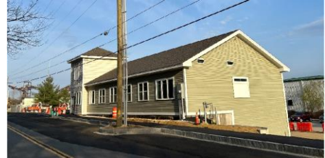
Inspection Services building is almost complete.
