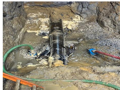
Washington St Water Main
