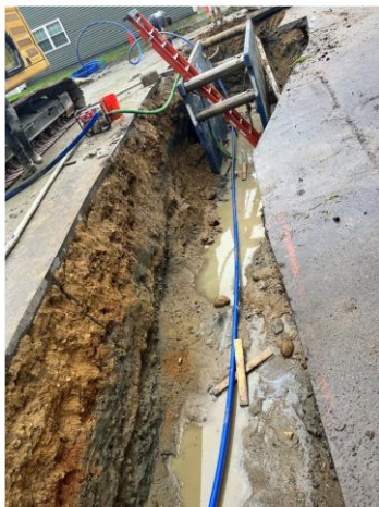
Water line, Cricket Brook
