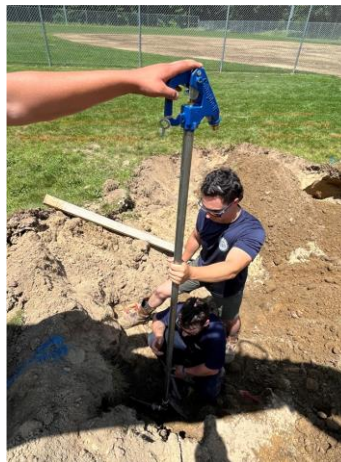
Yard hydrant installation at Guppy Park
