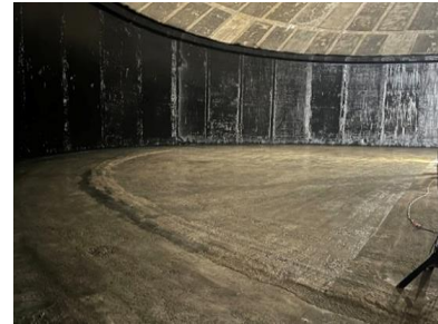
Garrison Hill Water Tank Interior Coating
