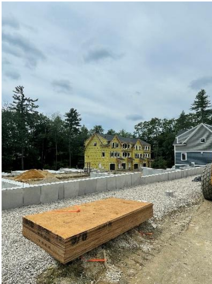
Lennox Drive Construction Site
