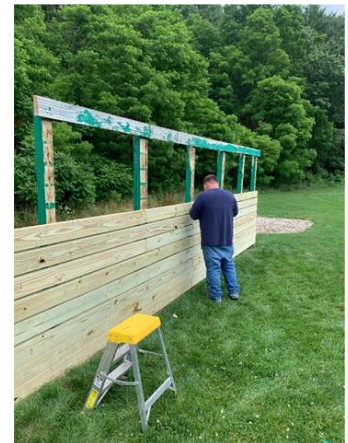
Kick wall at Shaw's Lane
