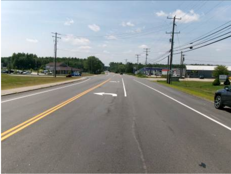
STREET SCENE – FRONT OF THE SUBJECT PROPERTY – CENTRAL PORTION Looking West on Knox Marsh Road - (7/25)
