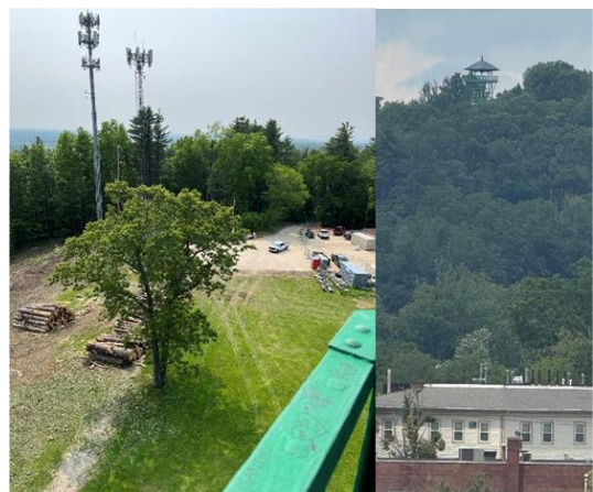
Garrison Hill Water Main Work site & Improved Tower Visibility
