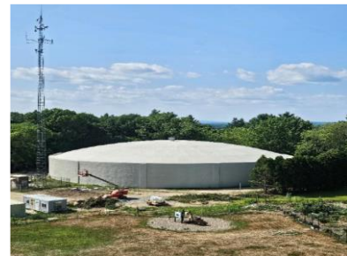
Garrison Hill Water Tank
