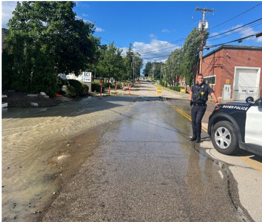
Broadway water main break
