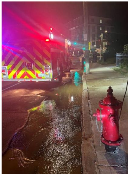
Central Ave service leak
