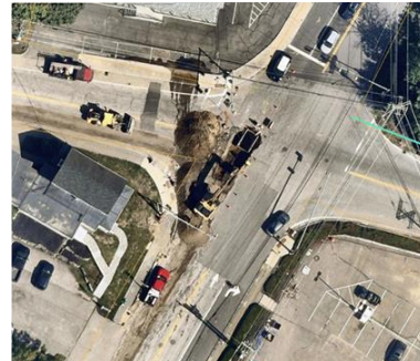
Water main installation work at the intersection of Oak St. and Broadway.
