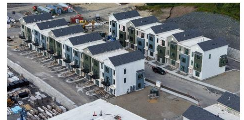
Residential Build Overview
