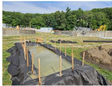
Support Nails at the third Secondary Clarifier
