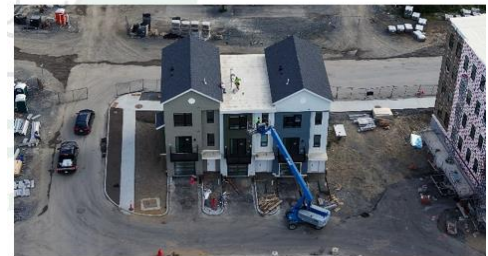
Residential Unit Construction
