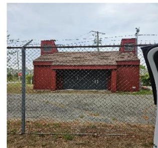
Wentworth Terrace Pump Station
