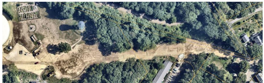
New Watermain installation from the Garrison Tank to Oak Street
