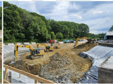
Third Secondary Clarifier Project Dig
